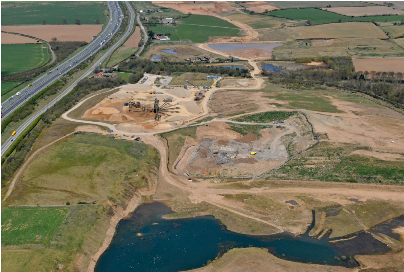
Aerial Photograph of the proposed site
